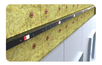
VFB 60/60- Product width across cavity 16mm up to 75mm wide, directly faced fixed, no additional pigtails required.
